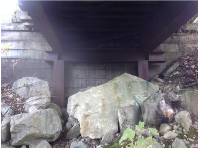
Right Bank Abutment when facing downstream
