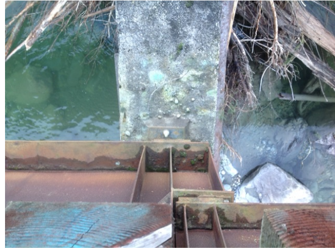
span 2 pier 2 connection typical
