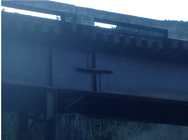
span 1 - span 2 connection
