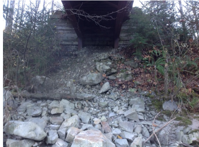
Left Bank Abutment when facing downstream
