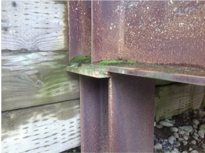
left bearing typical
