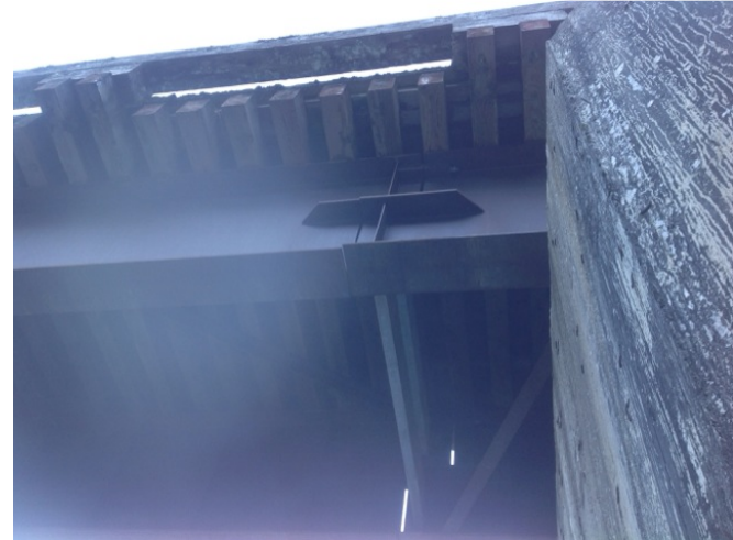
span 1 - span 2 connection
